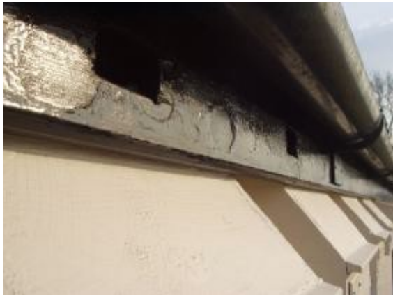
Holes cut in the facing boards let the Swifts reach their nests in the eaves of this chapel Photo © Mark Glanville
